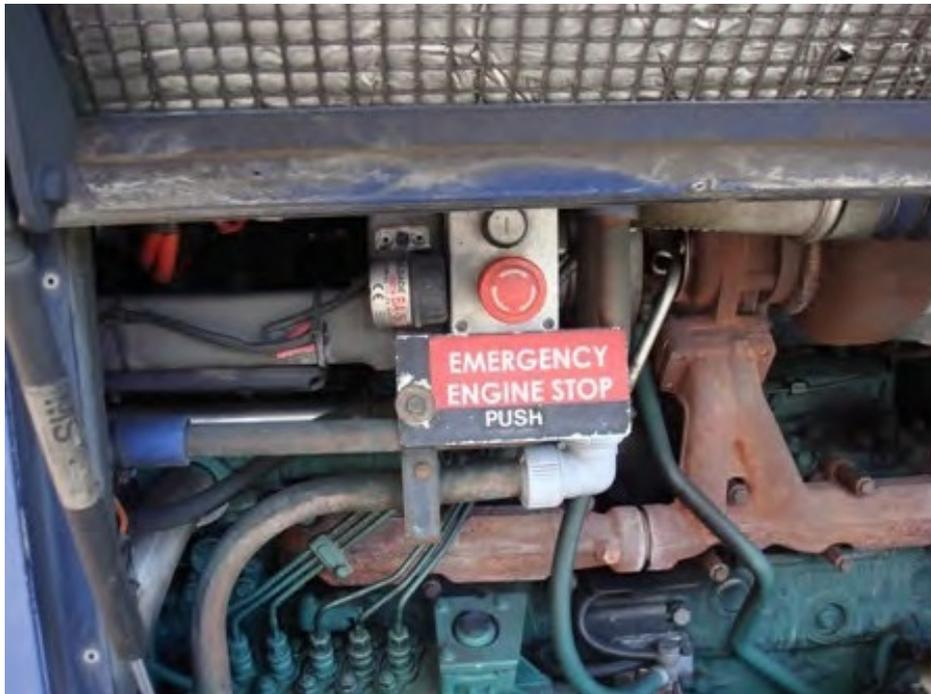
You can see in the pictures once you have opened the hatch there is a simple isolation button that locks, so once activated the engine can not be restarted until it has been reset.
